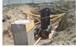
Installation of the special separator
